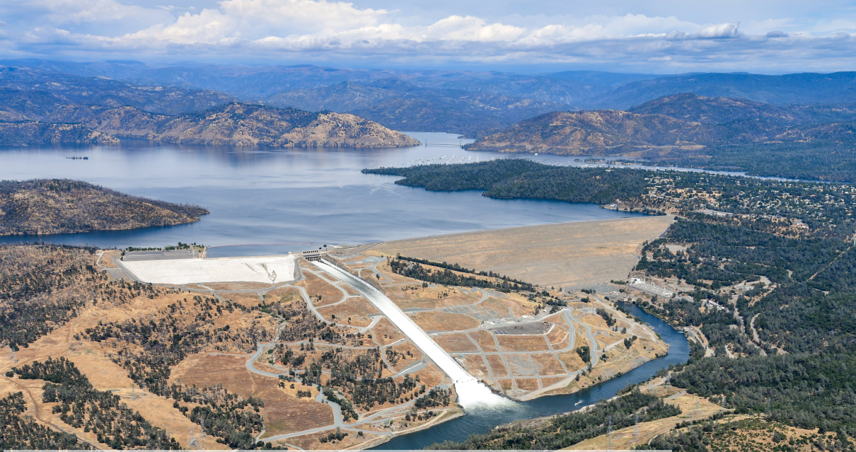
[ The Oroville embankment dam. By California Department of Water Resources. Public Domain, via Wikipedia. ]
